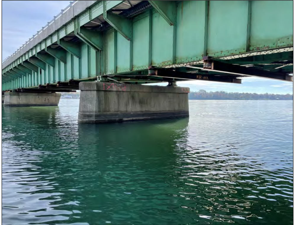
Pier 1w, west elevation
