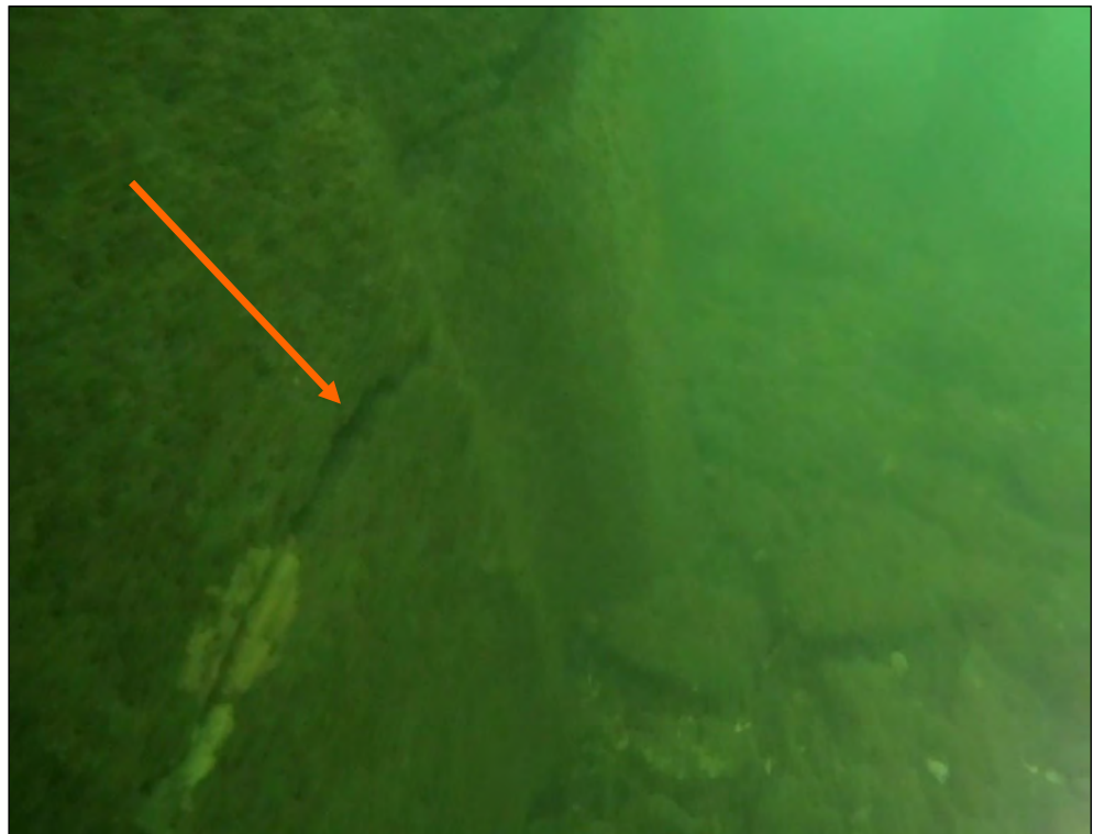
Pier 5w, open crack in footing, typical west and east elevations
