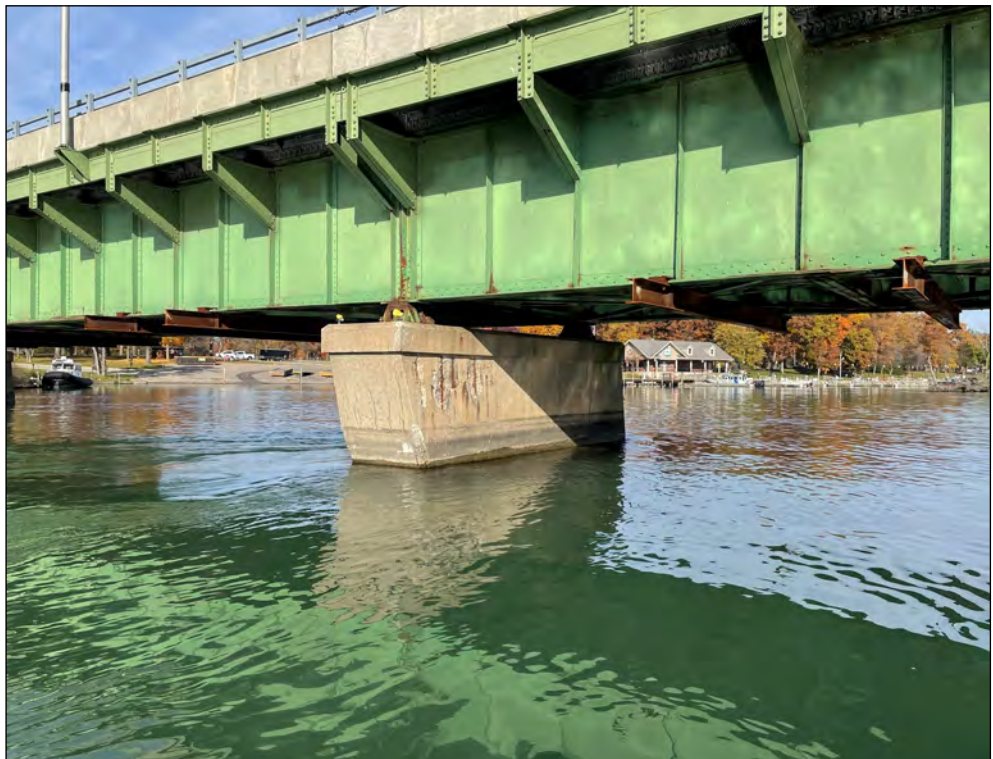
Pier 2w, east elevation
