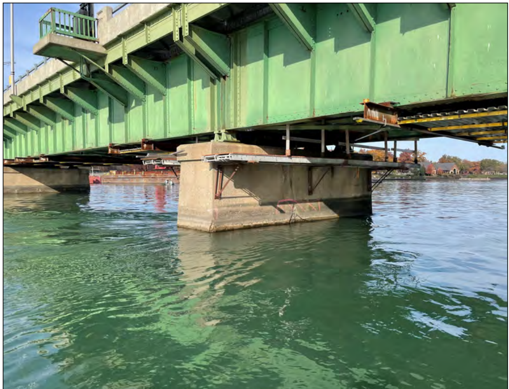
Pier 7w, east elevation
