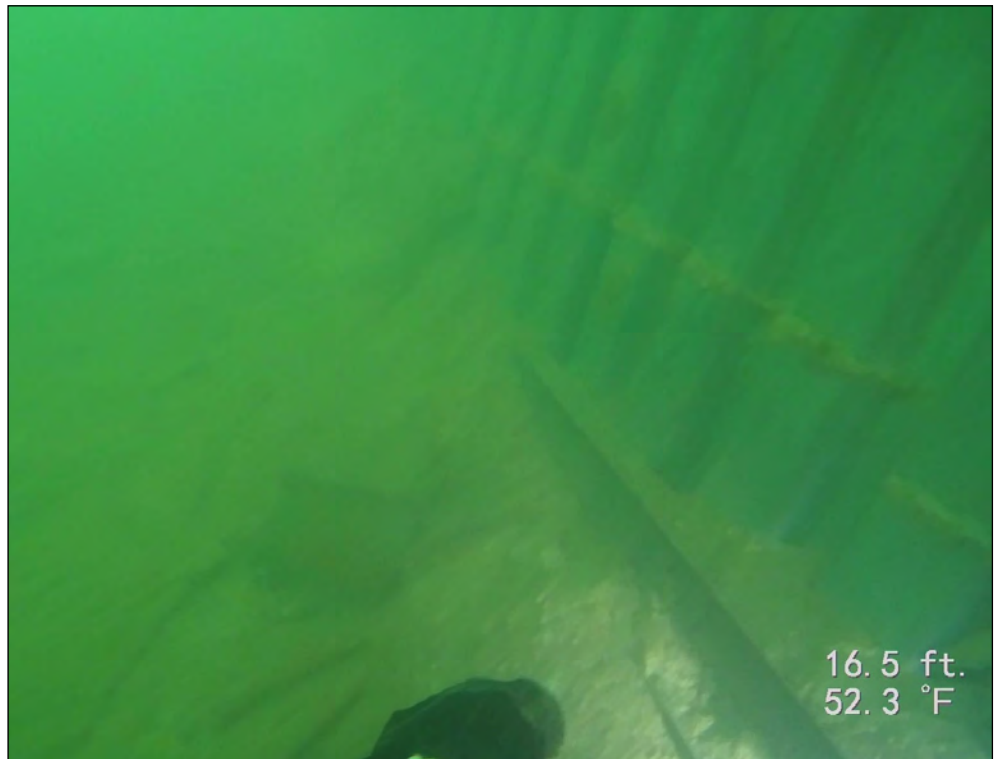
Pier 8w, steel sheeting and steel walers at channel bottom, typical
