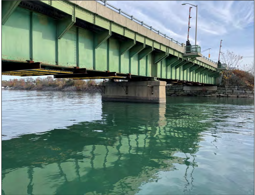
Pier 11w, west elevation
