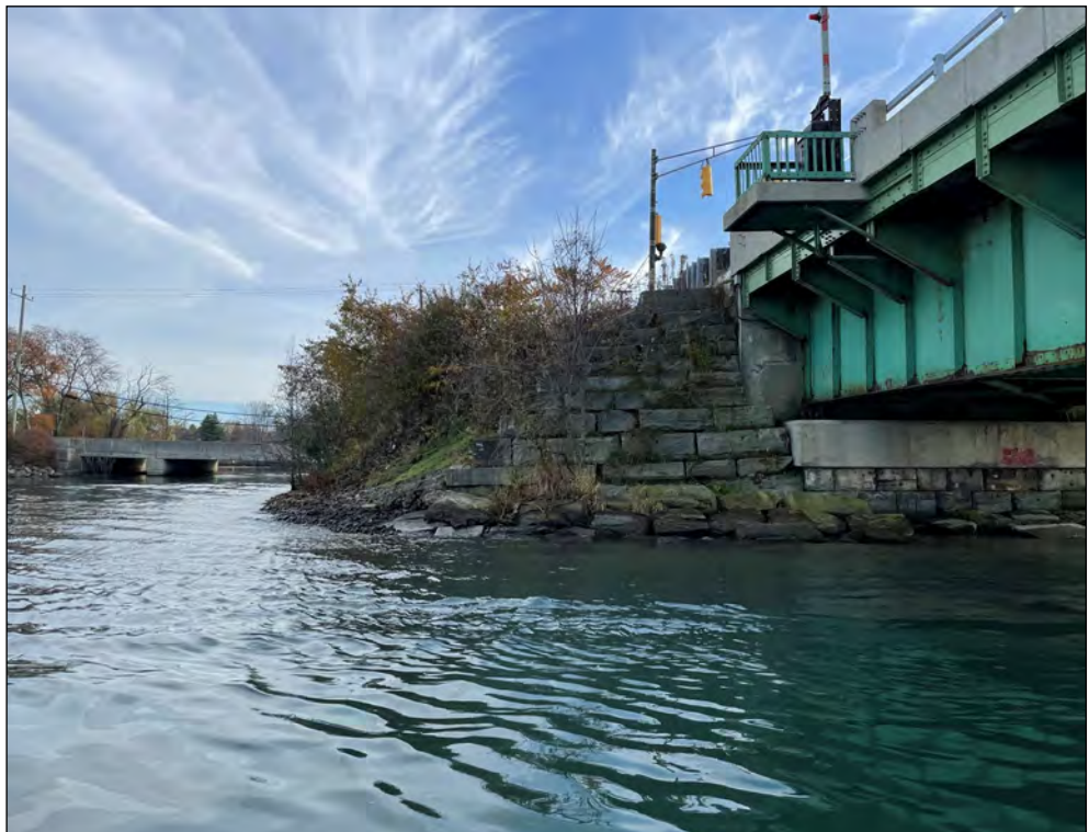
Northeast channel bank
