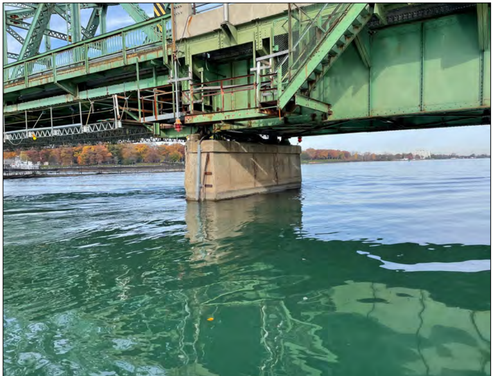
Pier 10w, east elevation
