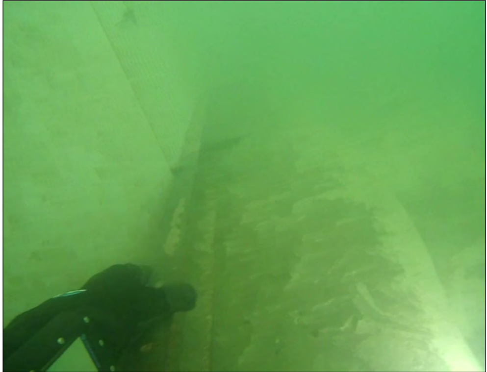
Pier 6w, grout bags and vinyl sheeting at channel bottom, typical
