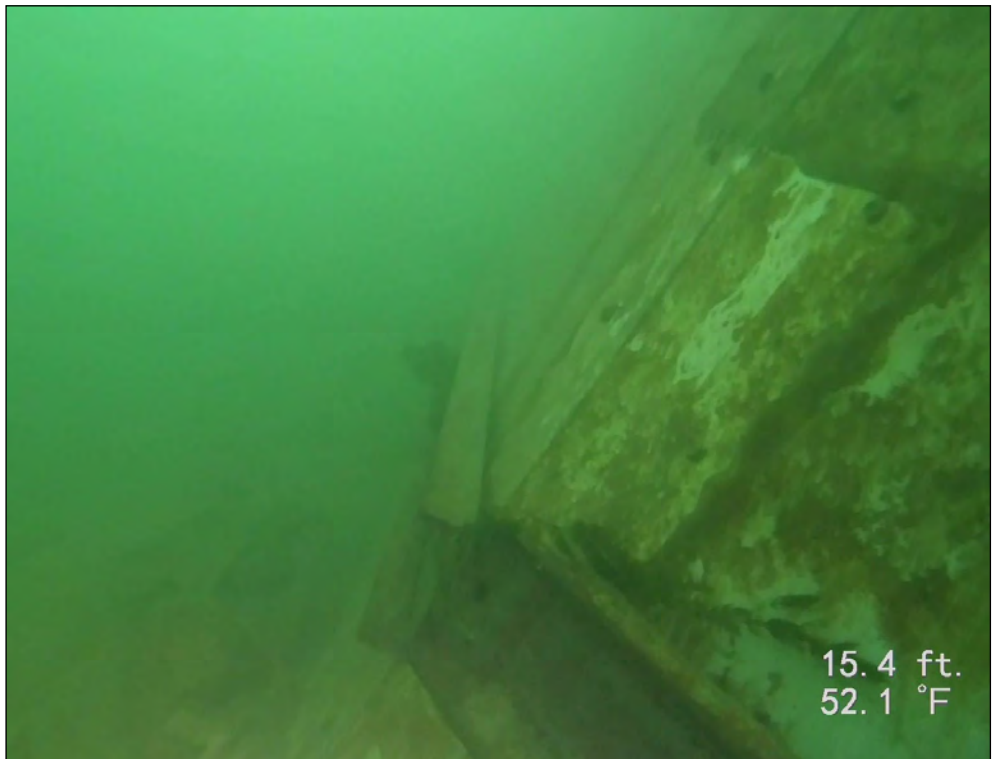
Pier 10w, vinyl sheeting and steel walers, typical
