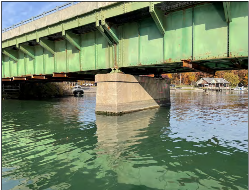
Pier 1w, east elevation
