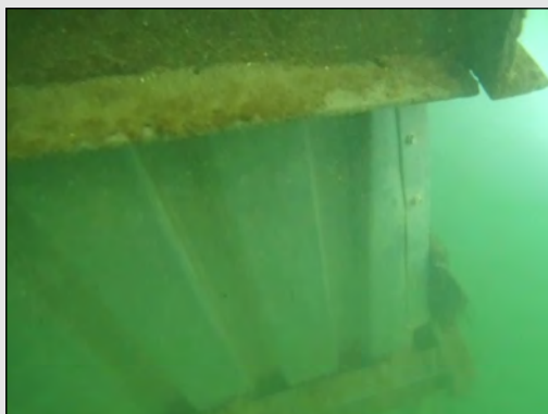
Steel stay-in-place forms and walers
