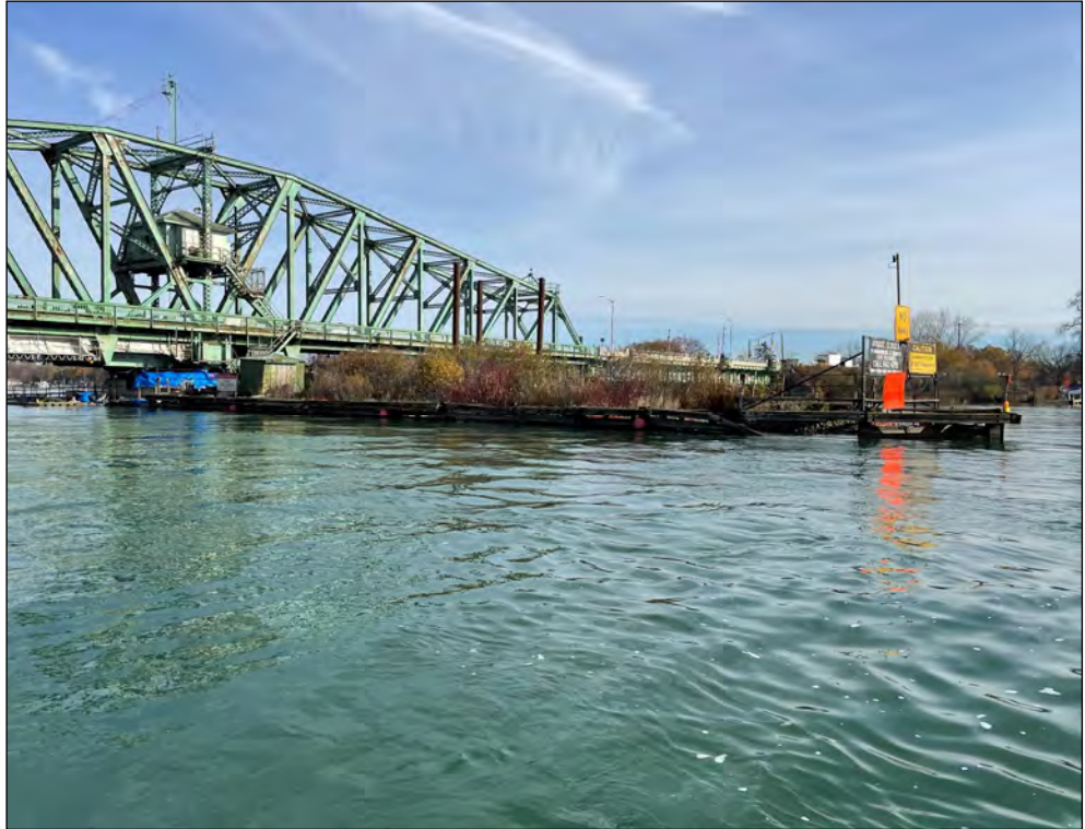
Pier 9w, southwest timber fender
