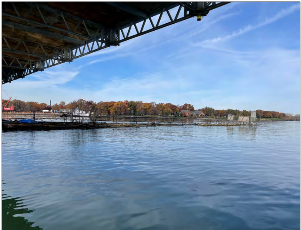
Pier 9w, northeast timber fender
