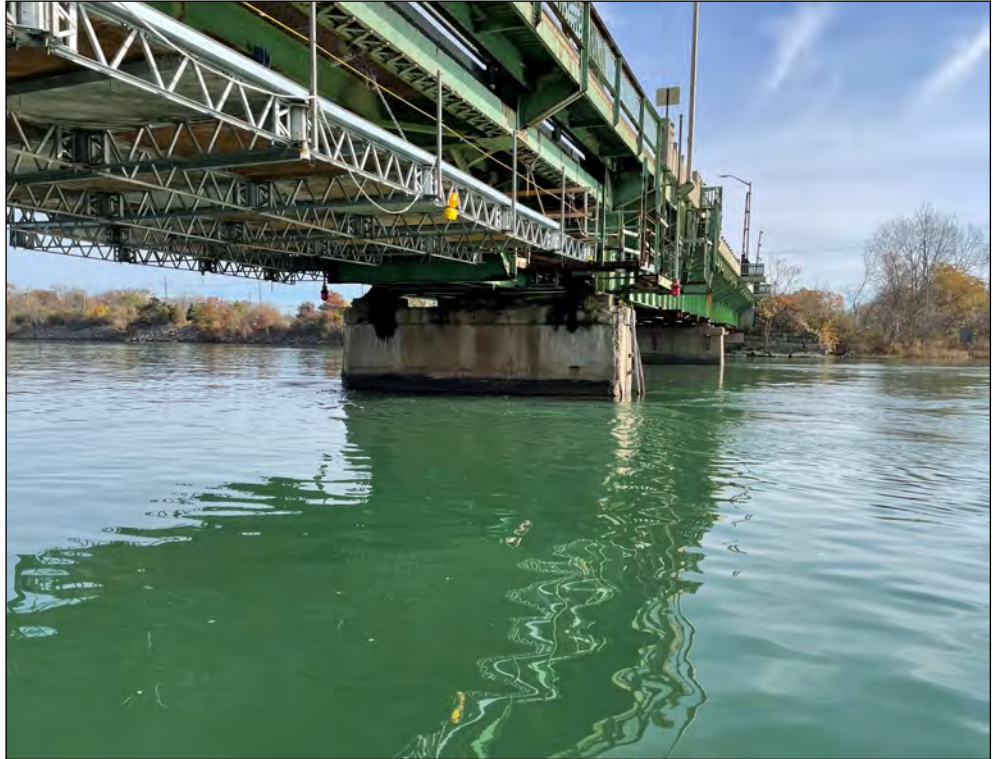
Pier 10w, west elevation
