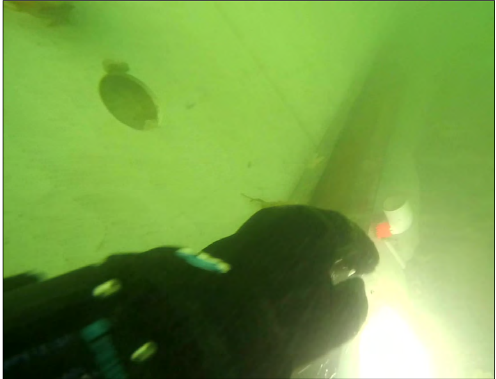
Pier 4w, vinyl sheeting at channel bottom, typical
