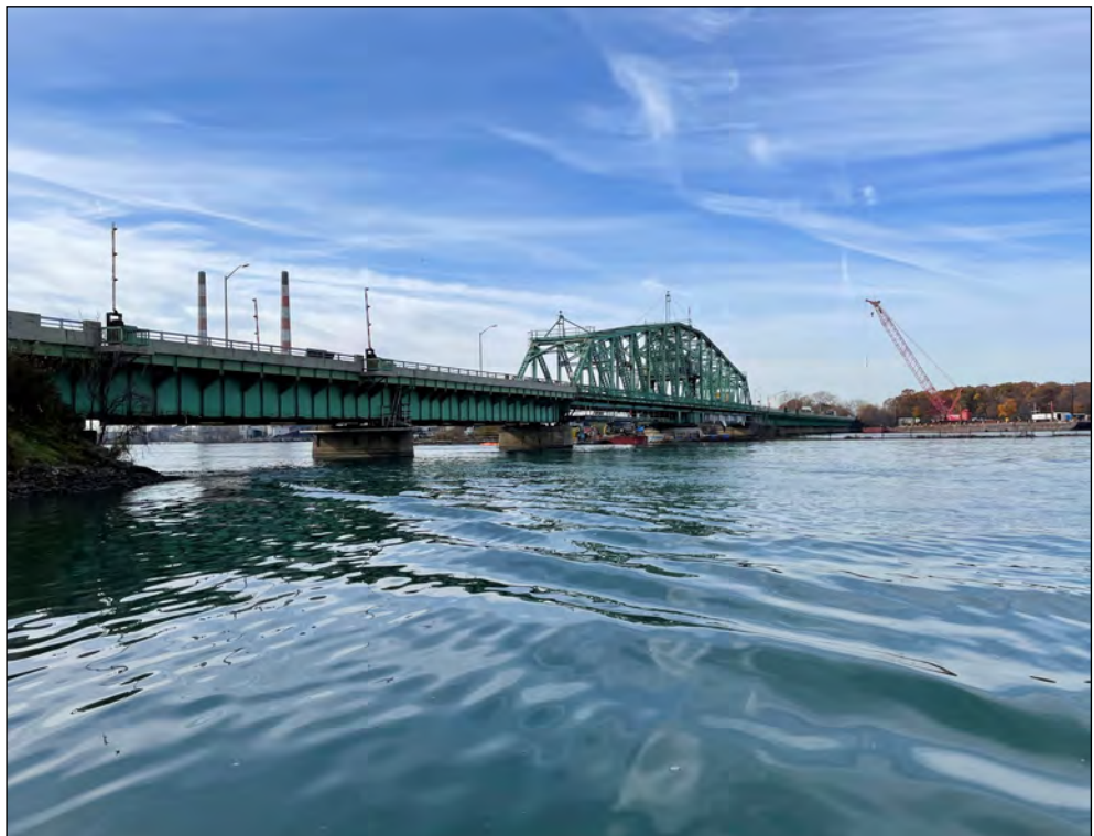
North elevation of bridge
