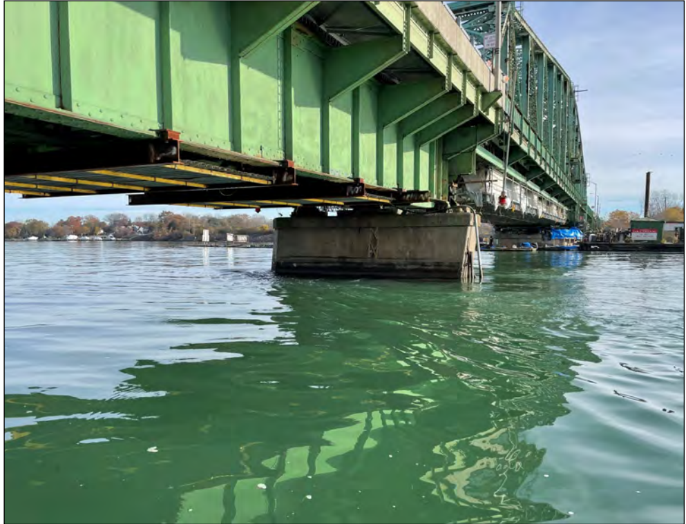
Pier 8w, west elevation
