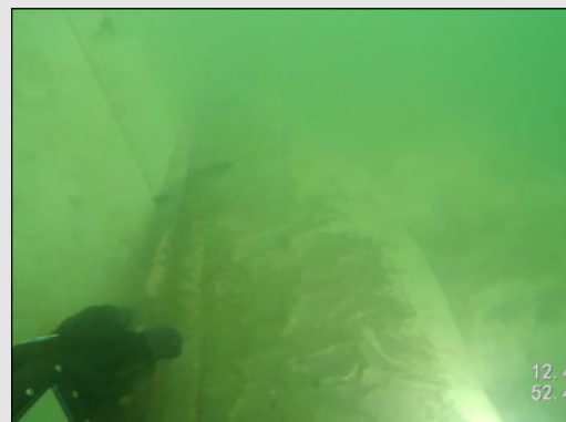
Grout bags and vinyl stay-place forms
