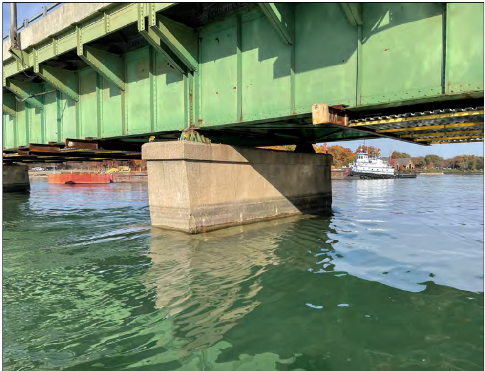
Pier 6w, east elevation
