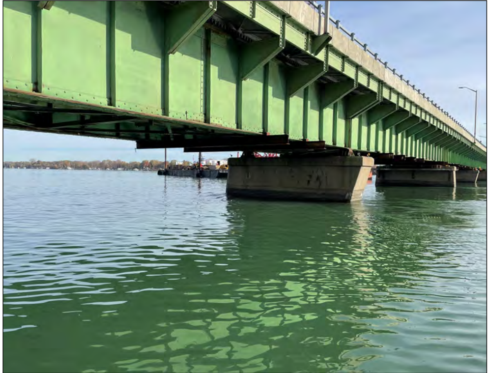
Pier 2w, west elevation
