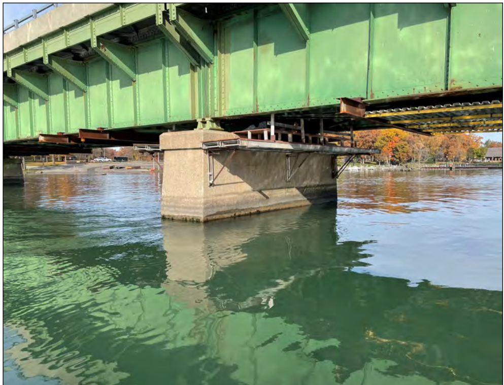
Pier 3w, east elevation
