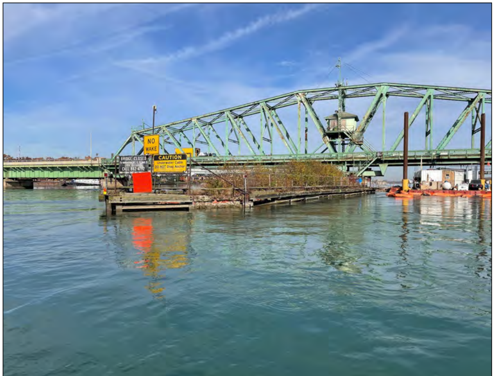
Pier 9w, southeast timber fender
