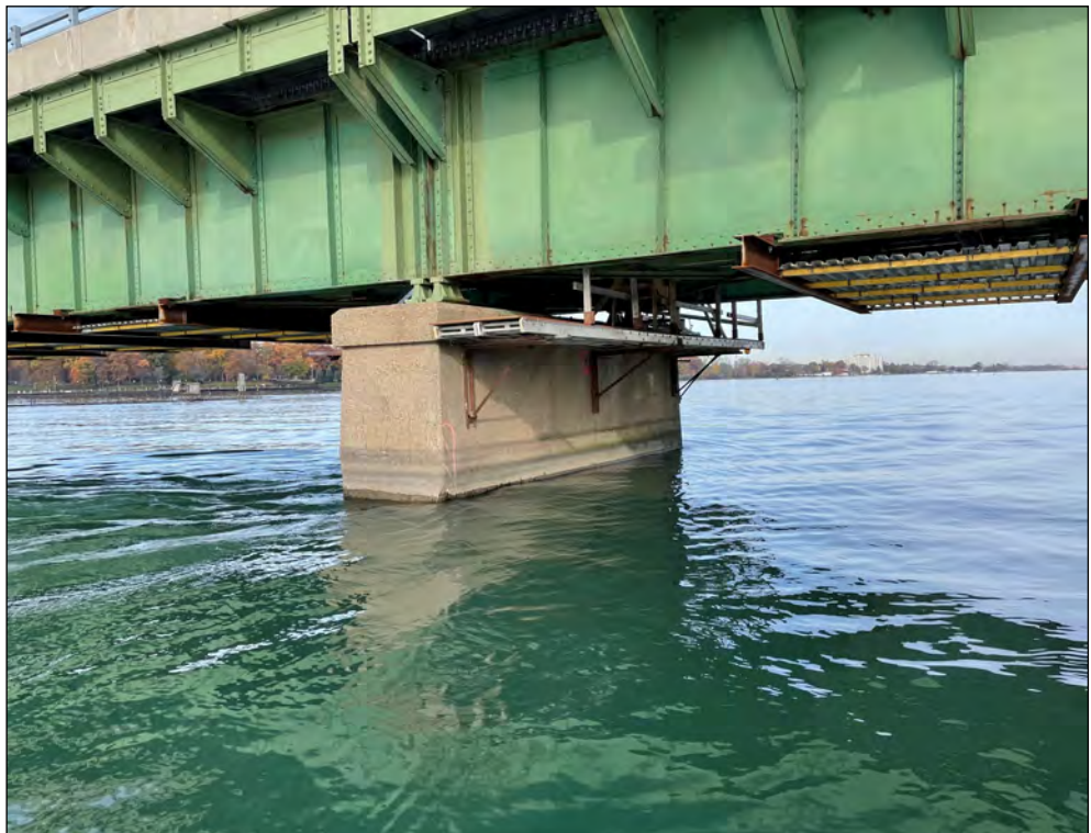
Pier 11w, east elevation
