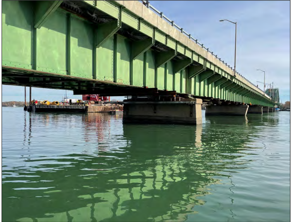
Pier 3w, west elevation
