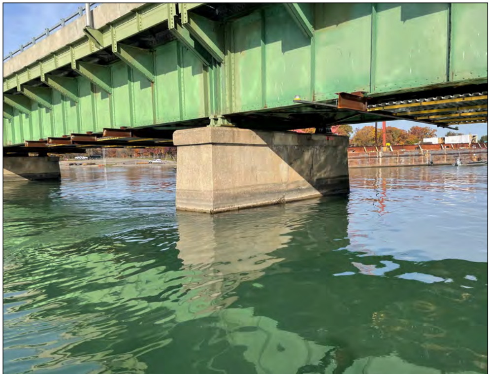
Pier 5w, east elevation
