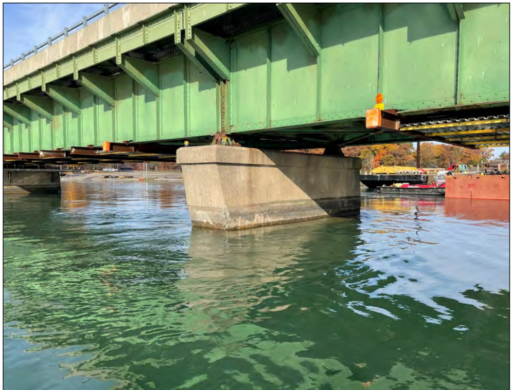
Pier 4w, east elevation
