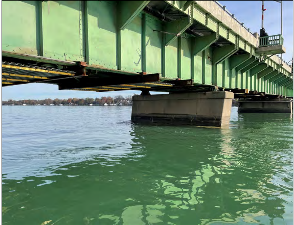
Pier 6w, west elevation
