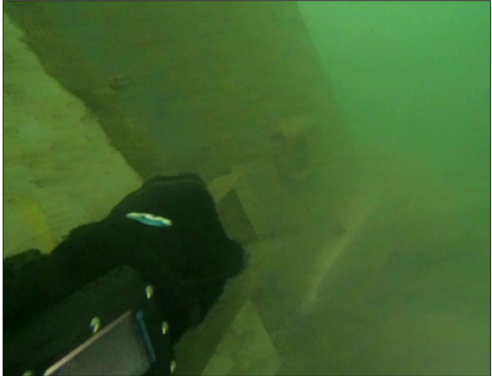
Pier 2w, steel ice breaker at channel bottom, typical
