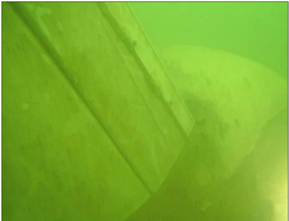
Pier 4w, vinyl sheeting and grout bags at channel bottom, typical
