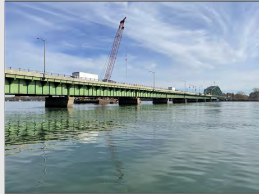
STR 12006 Grosse Ile Parkway over Trenton Channel Wayne County
