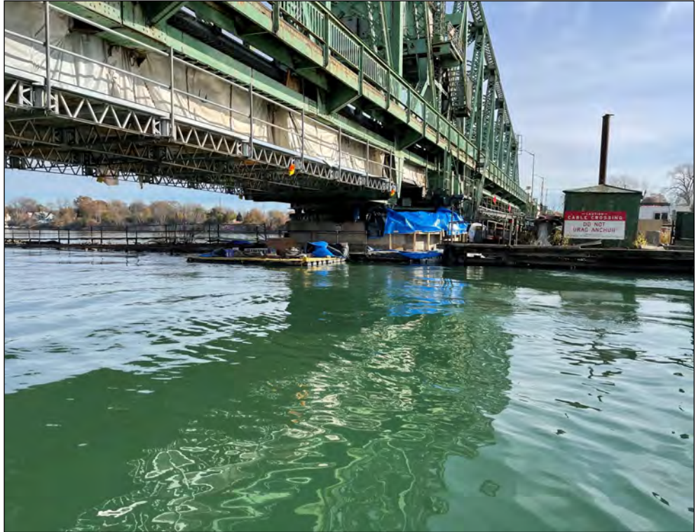
Pier 9w, west elevation
