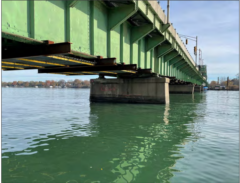
Pier 5w, west elevation
