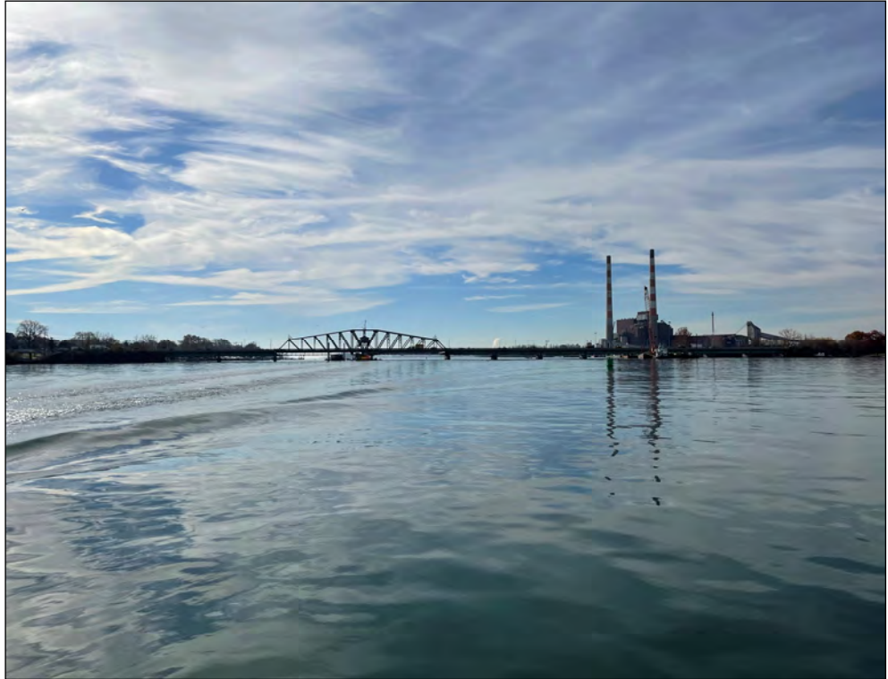
North elevation of bridge
