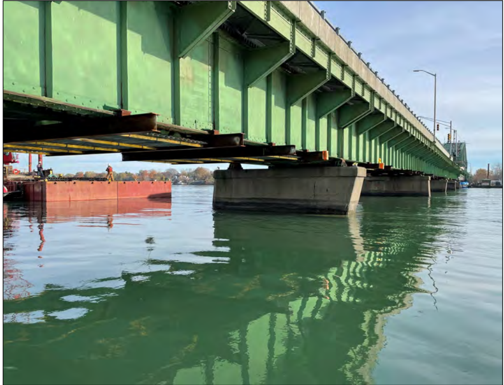
Pier 4w, west elevation
