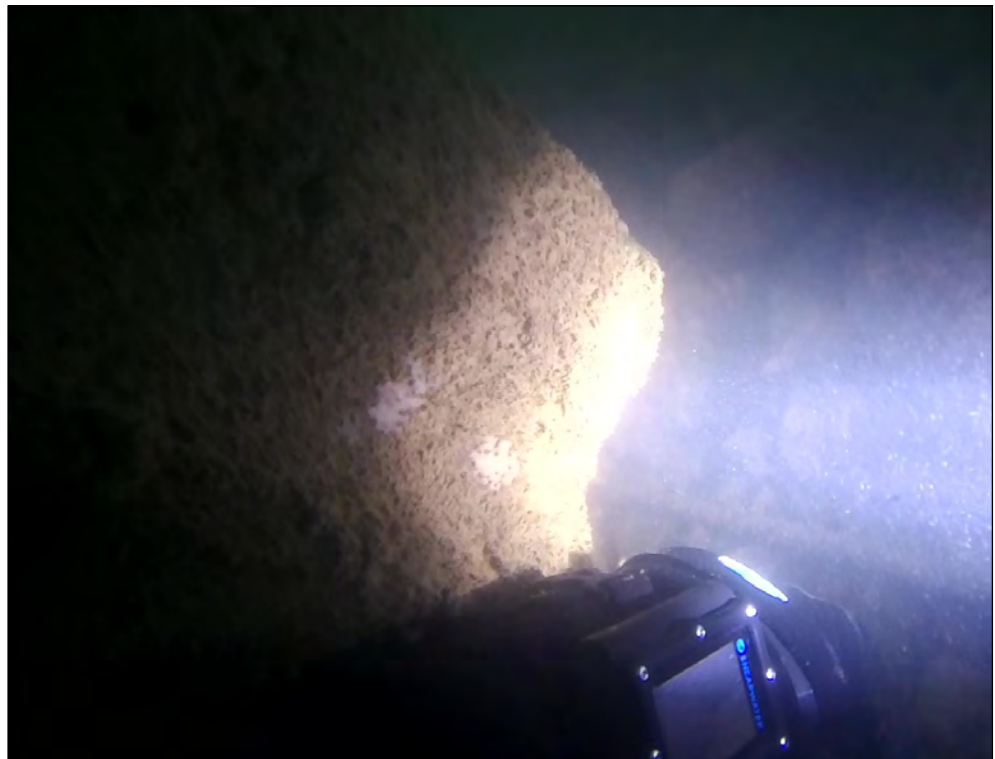
Pier 3w, typical condition of exposed footing
