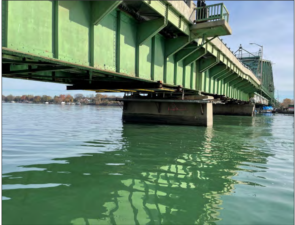
Pier 7w, west elevation
