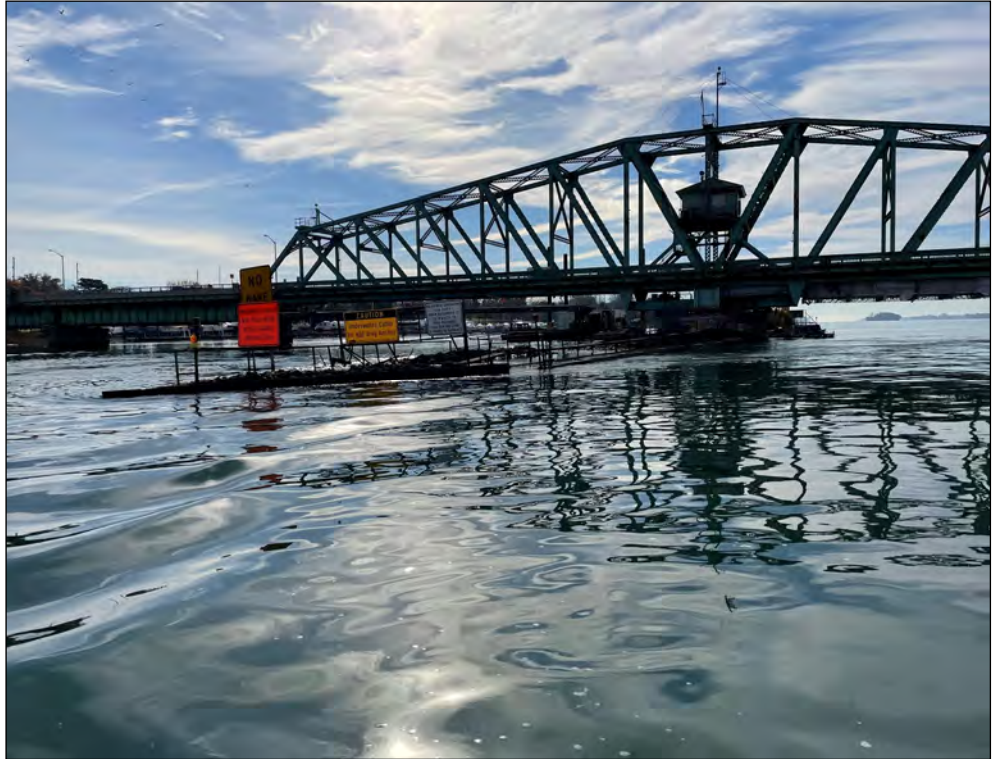
Pier 9w, northwest timber fender
