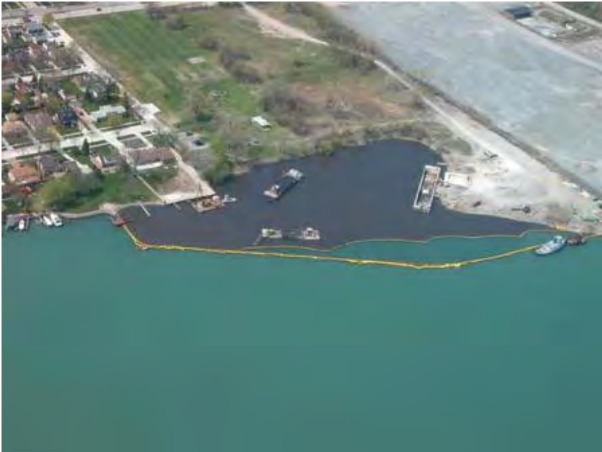
Photo: Detroit River Clean up Effort
