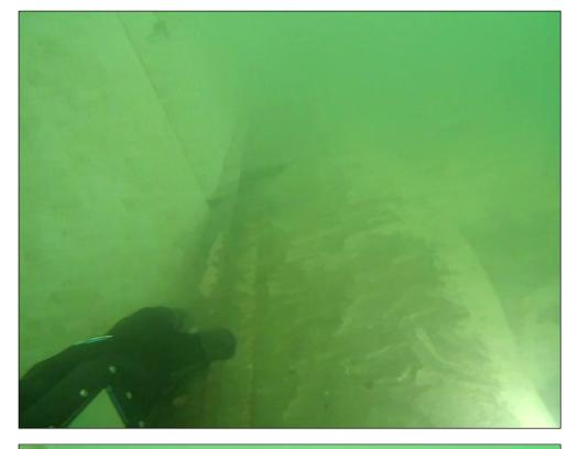
Pier 6w, corner of vinyl sheeting, steel walers and grout bags at channel bottom, typical
