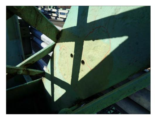
Span 10w, south truss, north gusset, vertical  $U_6$  -  $L_6$  section loss
