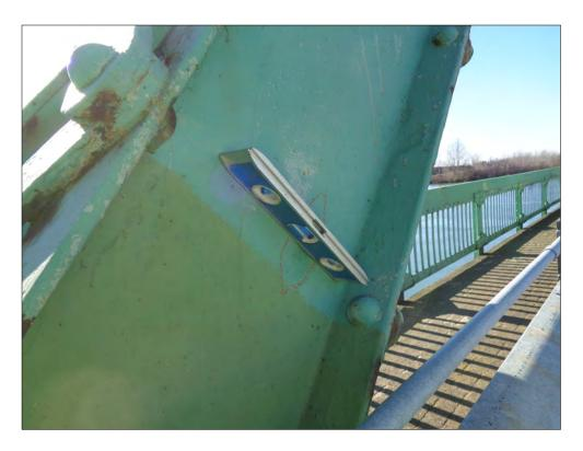
Span 9w, south truss, north face, diagonal  $U_2 - L_3$ section loss
