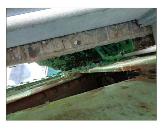
Span 10w, north truss, north face, diagonal  $L_{\theta}$  -  $U_{I}$  section loss
