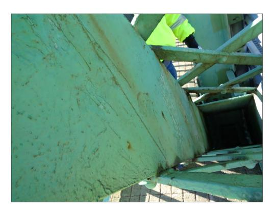
Span 10w, south truss, north face, diagonal  $U_4$  -  $L_3$ section loss
