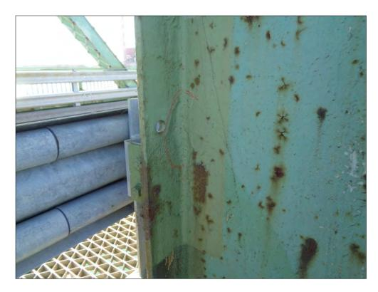
Span 10w, north truss, south face, diagonal  $U_1$  -  $L_2$  section loss
