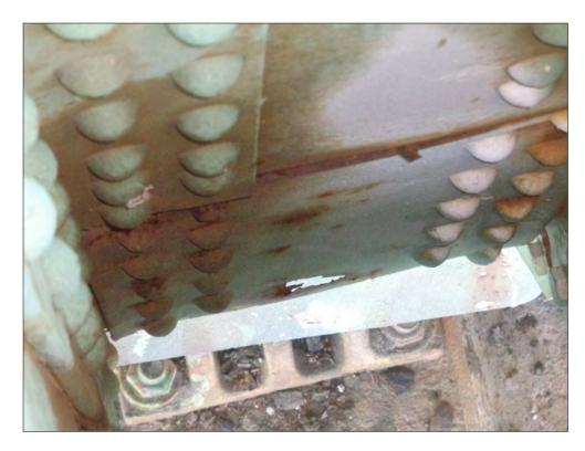
Span 9w, north truss, east face, web, vertical  $L_1$  -  $U_1$ section loss
