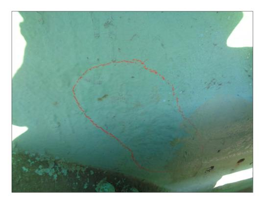
Span 9w, north truss, south face, diagonal  $U_2$  -  $L_3$ section loss
