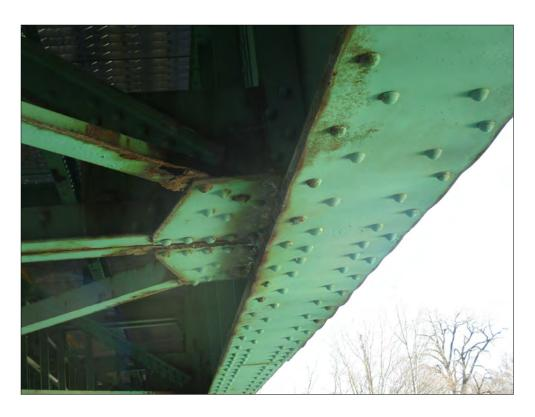
Span 11w, north girder, section loss at floorbeam 3w, 4w
