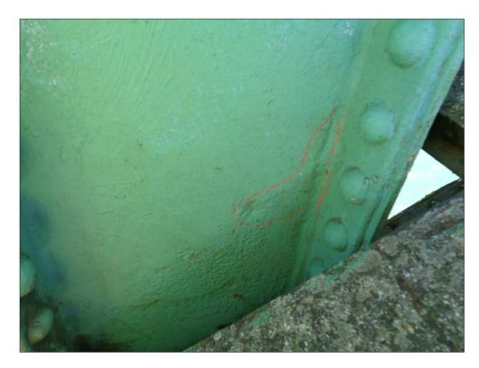
Span 9w, north truss, north face, diagonal  $U_5$  -  $L_6$ section loss
