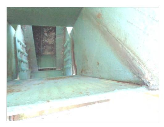
Span 10w, south truss, north face, diagonal  $U_2$  -  $L_1$  section loss
