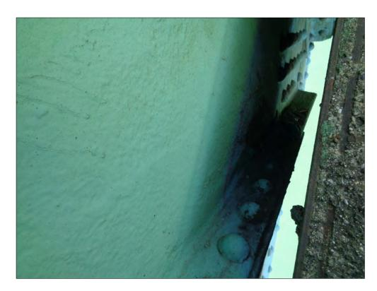
Span 10w, north truss, north face, diagonal  $U_4$  -  $L_3$ section loss
