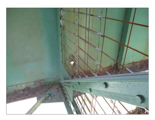
Span 1w, south girder, floorbeam 2w, 5" x 5" hole in web
