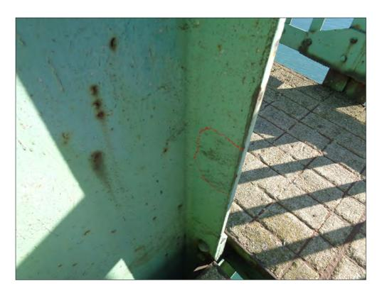
Span 10w, south truss, north face, diagonal U<sub>3</sub> - L<sub>2</sub> section loss
