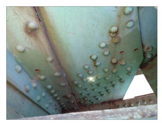
Span 10w, south truss, north face, diagonal  $U_I$  -  $L_\theta$  section loss
