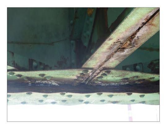
Span 3w, north girder, section loss at floorbeam 3w, 4w
