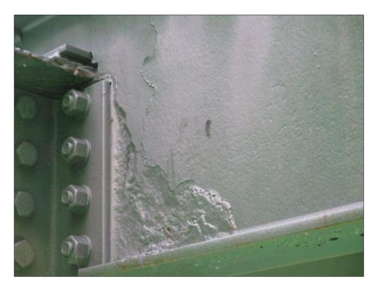
Span 2w, floorbeam 2w, bay 1w, stringer 2s, web loss of section
