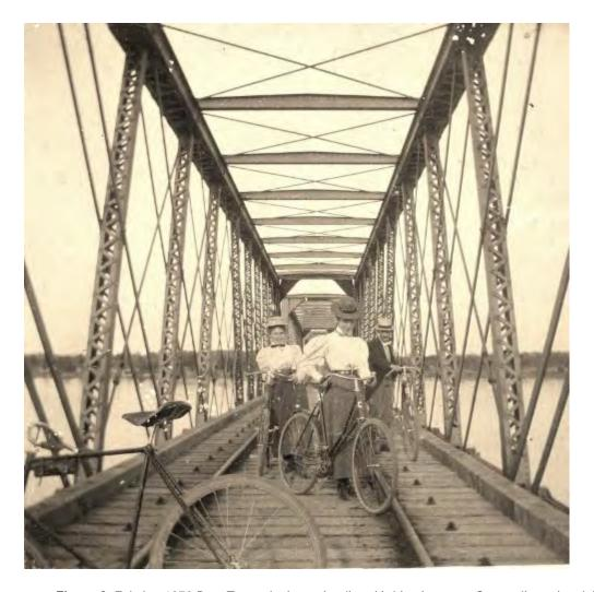
Figure 2 Existing 1873 Post Truss single-track railroad bridge between Grosse Ile and mainland Michigan
