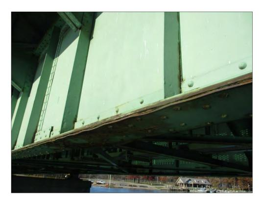
Span 4w, north girder, section loss at floorbeam 3w, 4w
