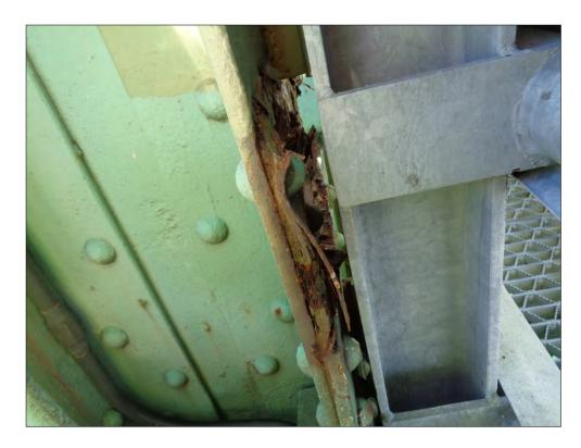
Span 9w, north truss, lower gusset, south plate, L<sub>0</sub>, holes
