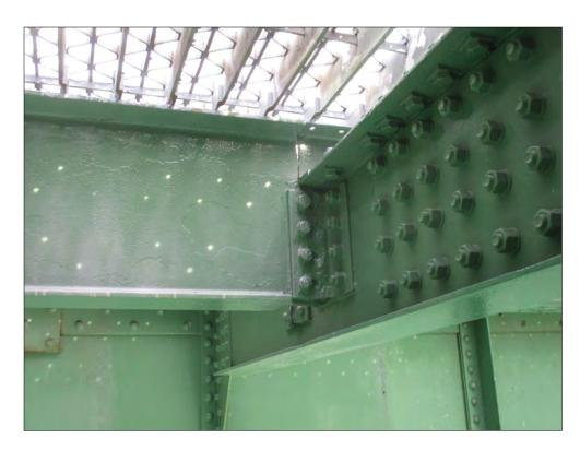
Span 7w, floorbeam 4w, Stringer/ floorbeam connection
