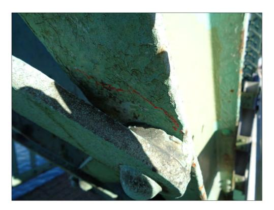
Span 9w, north truss, north face, diagonal  $U_3$  -  $L_4$ section loss
