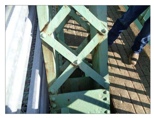
Span 10w, south truss, south face, diagonal  $U_2$  -  $L_1$  section loss
