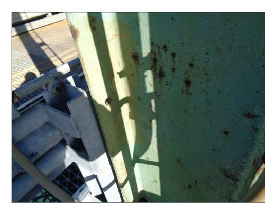
Span 10w, south truss, north face, vertical  $U_1$  -  $L_1$  section loss
